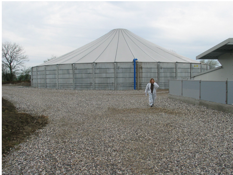
Figure 6. Slurry tank with tent for limiting the ammonia emission from storages
